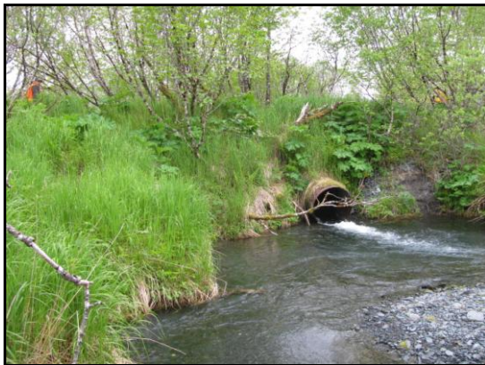
This old military culvert above Buskin Lake was determined to be inhibiting fish passage and is now planned for removal, the orange vests in the photo mark the approximate excavation width (left). Upstream of the same culvert, David Wigglesworth and Bill Rice, USFWS, stretch a tape demonstrating the natural stream width at high water (right).
