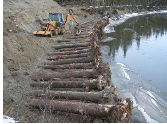
Root wads being installed for restoration project
