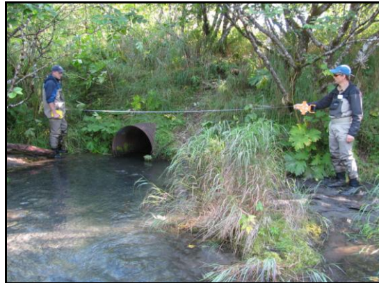
This old military culvert above Buskin Lake was determined to be inhibiting fish passage and is now planned for removal, the orange vests in the photo mark the approximate excavation width (left). Upstream of the same culvert, David Wigglesworth and Bill Rice, USFWS, stretch a tape demonstrating the natural stream width at high water (right).
